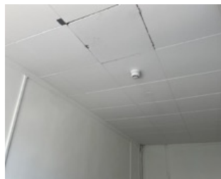
Asbestolux ceiling tiles
