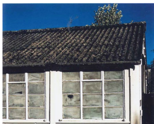
Asbestos cement roof
