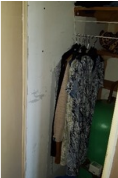
Asbestolux in a cupboard wall
