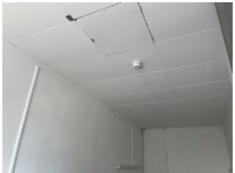
Asbestolux ceiling tiles
