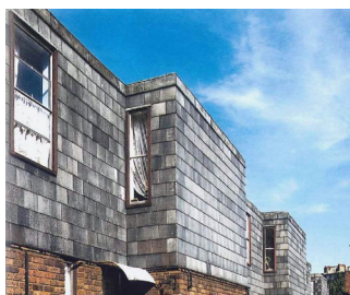
Asbestos cement tiles
