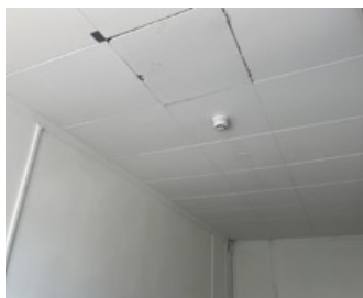
Asbestolux ceiling tiles
