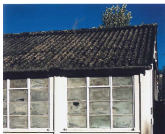
Asbestos cement roof
