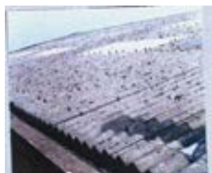
Asbestos corrugated roof
