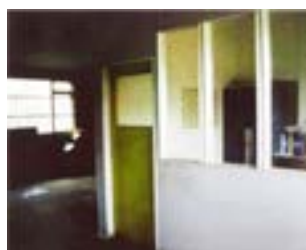
Asbestos insulating boards
