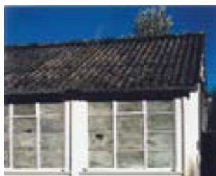
Asbestos cement roof
